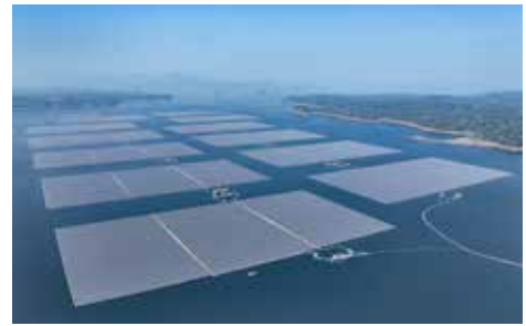
Indonesia-ANDRE HIDAYAT-Cirata Floating Solar Power Plant
