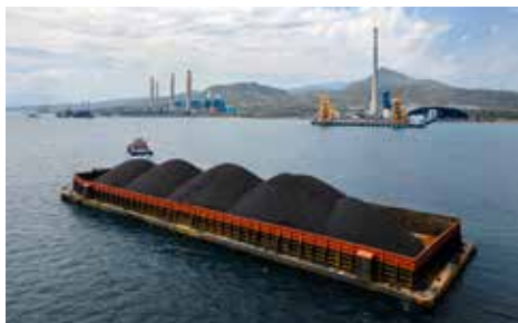
Indonesia-Anom Harya-Indonesian Power Plant
