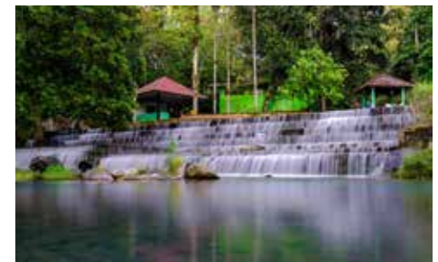
Indonesia-YUYUN RND-Sesaot Dam at Lombok
