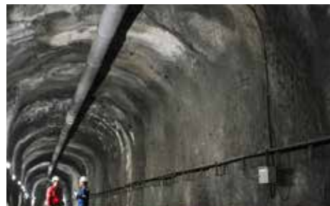
Indonesia-WIRAWAN SUHIRMAN- Working Tunnel Hydropower-.jpeg
