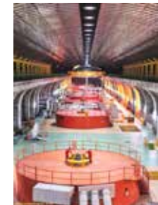
Indonesia-WIRAWAN SUHIRMAN- Cirata Underground Powerhouse- jpeg
