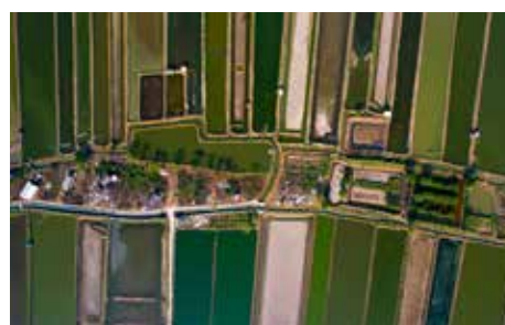
Indonesia-Soewignyo Koesnadi-Irrigation canal
