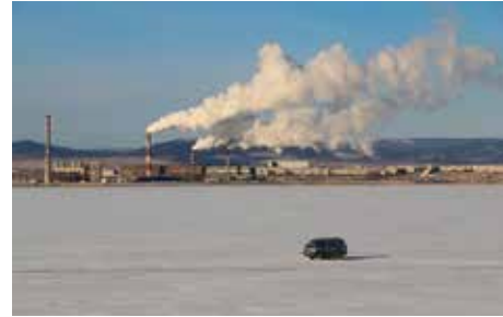
Argentina-Anna Perevozchikova- Water intake for heating plant
