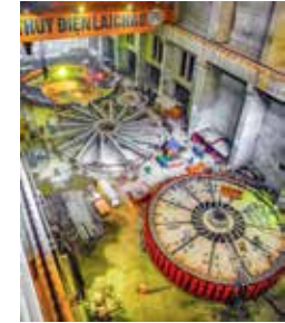
Vietnam-Van Dong Nguyen- assembling turbines at Lai Chau hyd
