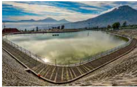
Indonesia-M. JEFFRY HANAFIAH- Temanggung Highlands Reservoir
