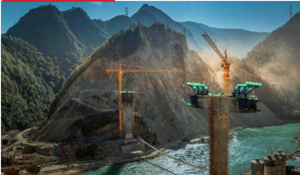
BRIDGE CONSTRUCTION Xiaoping Chen China
