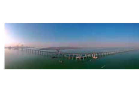
China-Yongling Sun-Coastal corridor under construction
