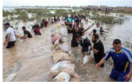
Iran (Islamic Republic of)-Ali Mohammadi-Dam construction
