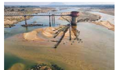
India-SUDIP SAHA-Tapping Sub surface water
