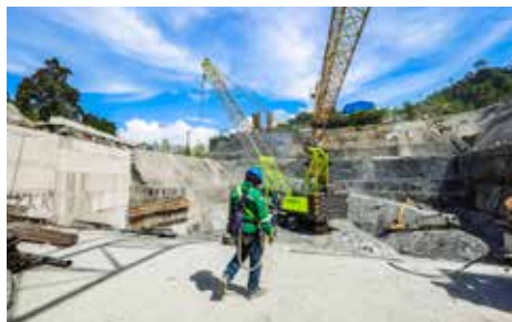
Indonesia-DIKYE ARIANI-Start tunnel excavation from above
