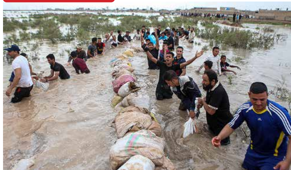
DAM CONSTRUCTION Ali Mohammadi Iran (Islamic Republic of)
