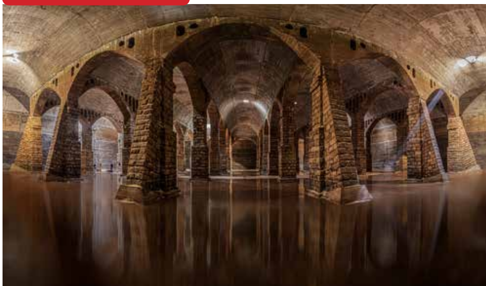
LUQA MALTA - NAVAL WATER RESERVOIR
