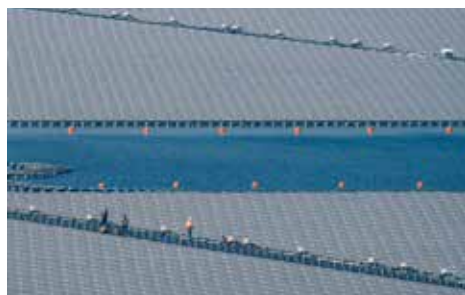
Indonesia-ANDRE HIDAYAT-Floating Solar Power Plant Workers
