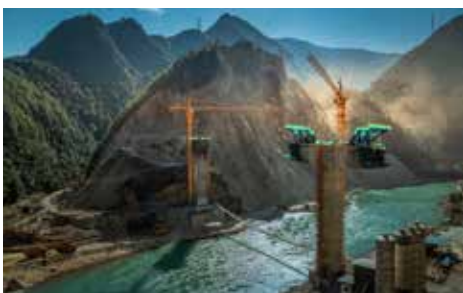
China-Xiaoping Chen-Bridge construction
