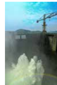
Indonesia-Dede Sudiana-Jatiluhur Hydroelectric Power Plant
