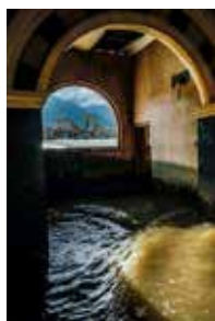
Indonesia-ICHSAN SAID-Construction of tsunami embankments
