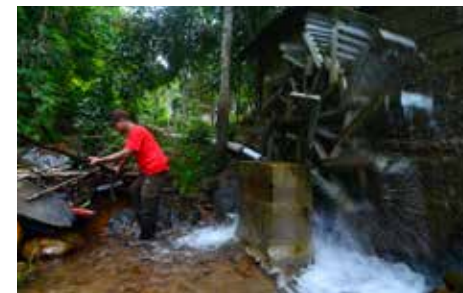
Indonesia-Saipullah-Hydroelectric Power Plant
