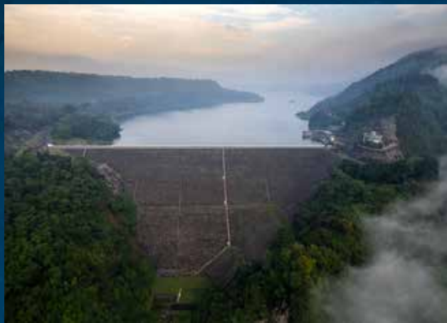
The Cirata hydro power plant ACCEPTED
