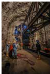
Indonesia-DIKYE ARIANI- Construction of hydroelectric power
