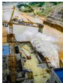
Vietnam-Van Dong Nguyen- construction site at Lai Chau hydro
