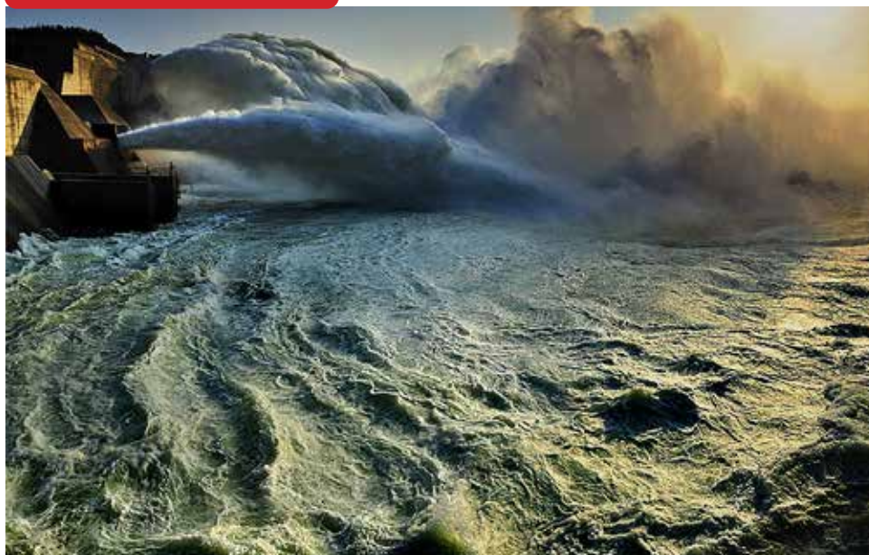
FLOOD DISCHARGE Yazhou Zhao China
