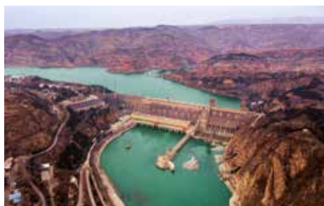
China-Xiujian Zhou-The Yellow River Green Dam
