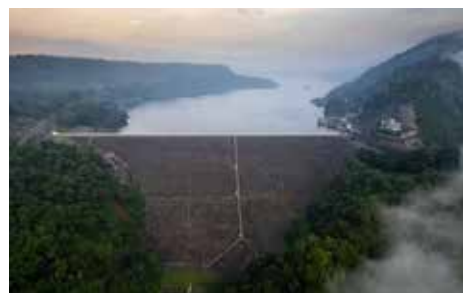
Indonesia-ISMAIL ABDUL MUTTALIB-The Cirata hydro power plant
