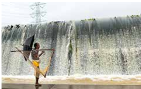
India-PIYALI MITRA-Check dam
