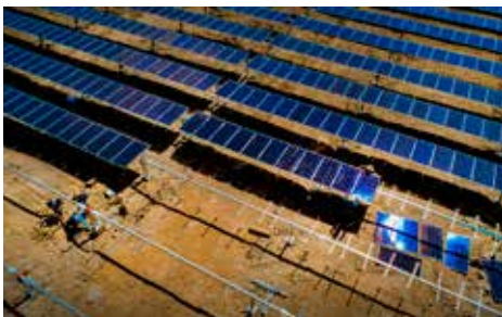
Vietnam-Van Dong Nguyen- construction of solar energy system
