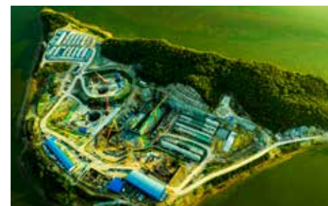
China-Jianning Wu-Water project of Pearl River Delta
