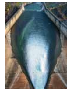
Indonesia-RIZAL ADI DHARMA-Jatigede Dam From Above
