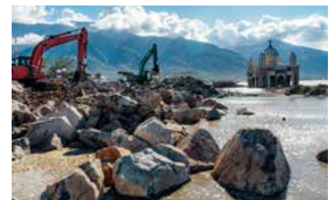
Indonesia-ICHSAN SAID-Construction of tsunami embankments-(1).jpg
