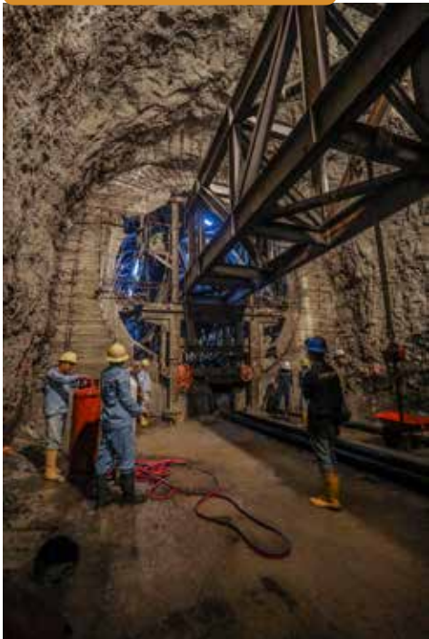
CONSTRUCTION OF HYDROELECTRIC POWER Dikye Ariani Indonesia
