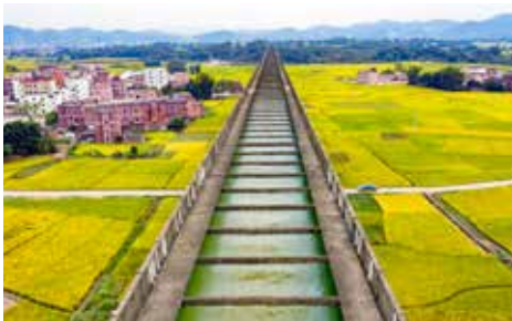
China-jianxing zhu-Rural Aqueduct -- Built in 1976, th
