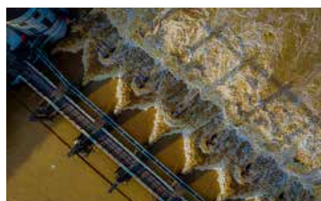
China-Jianning Wu-Ganzhutan Flood Discharge
